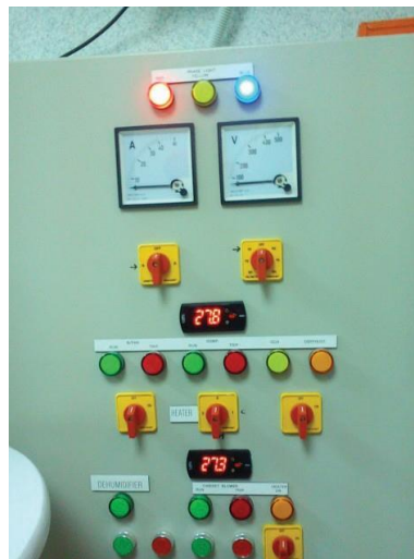
Figure 2: Environmental chamber main switch controller
