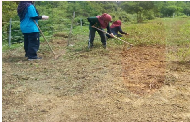
Figure 3.2: Site clearing activities in Agro Park, UMK Jeli
