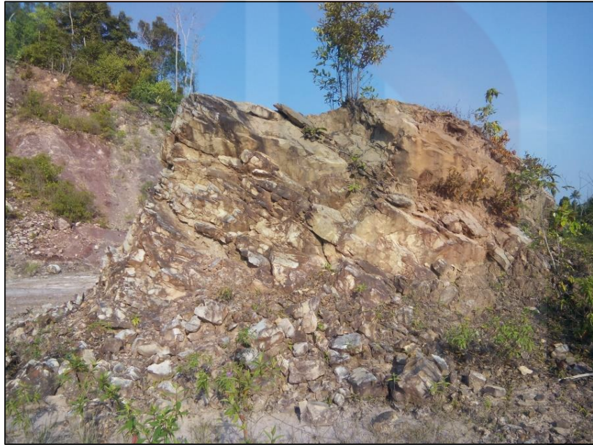
Figure 4.10: Biological weathering involves plant roots in study area.
