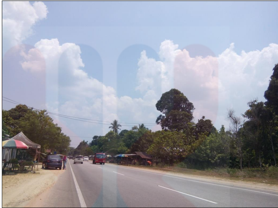
Figure 1.7: Paved roads connecting the study area with the nearby town (GPS: N 05°53'12.3" E 102°10'16.9")
