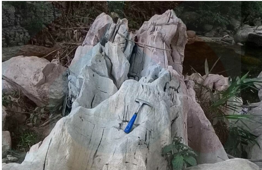
Figure 5.10 : Joints at location 3
