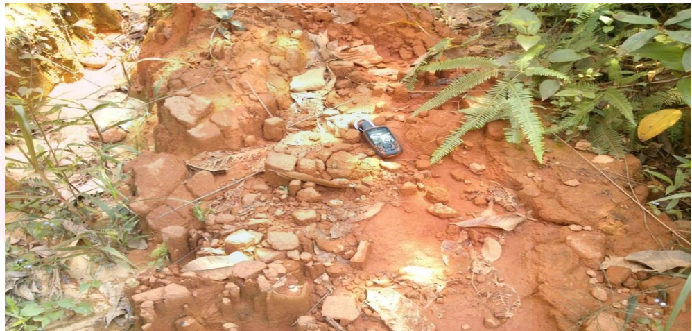
Figure 4.10: Chemical weathering (101°52'54.4'' E and 5°34'16.1'' N)
