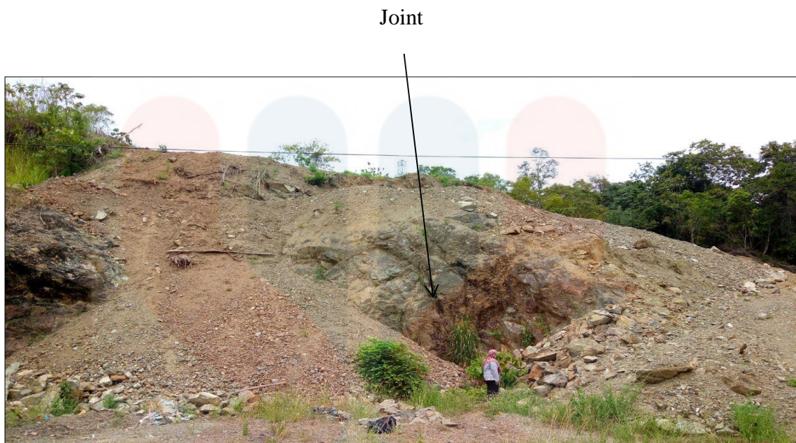
Figure 4.32: The joint on the rock of the andesite
