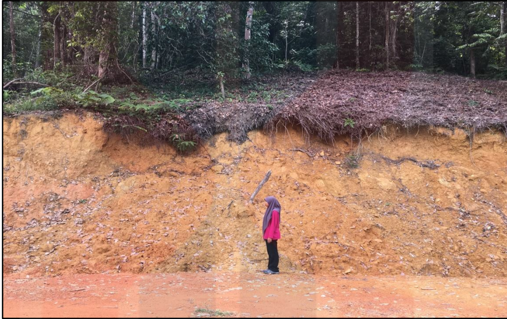
Figure 5.4: Slope failure at coordinate N 04°56'56.8 and E 102°03'19.5".
