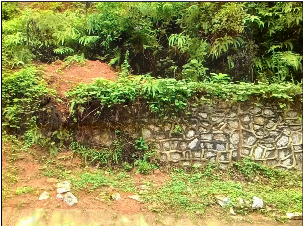
Figure 5.7 Stone pitching at location 1
