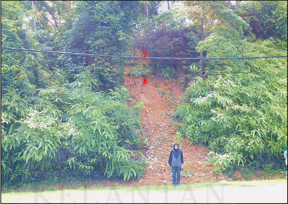
Figure 5.5 Slope failure at location 4
