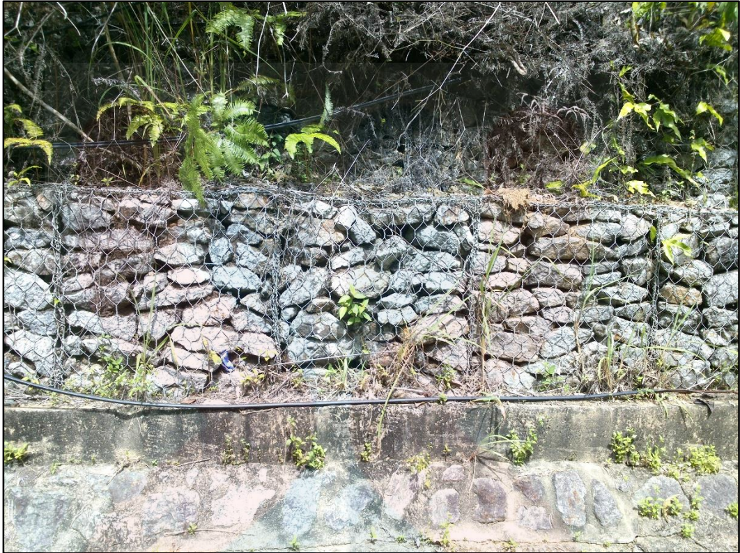
Figure 5.6 Gabion wall at location 3
