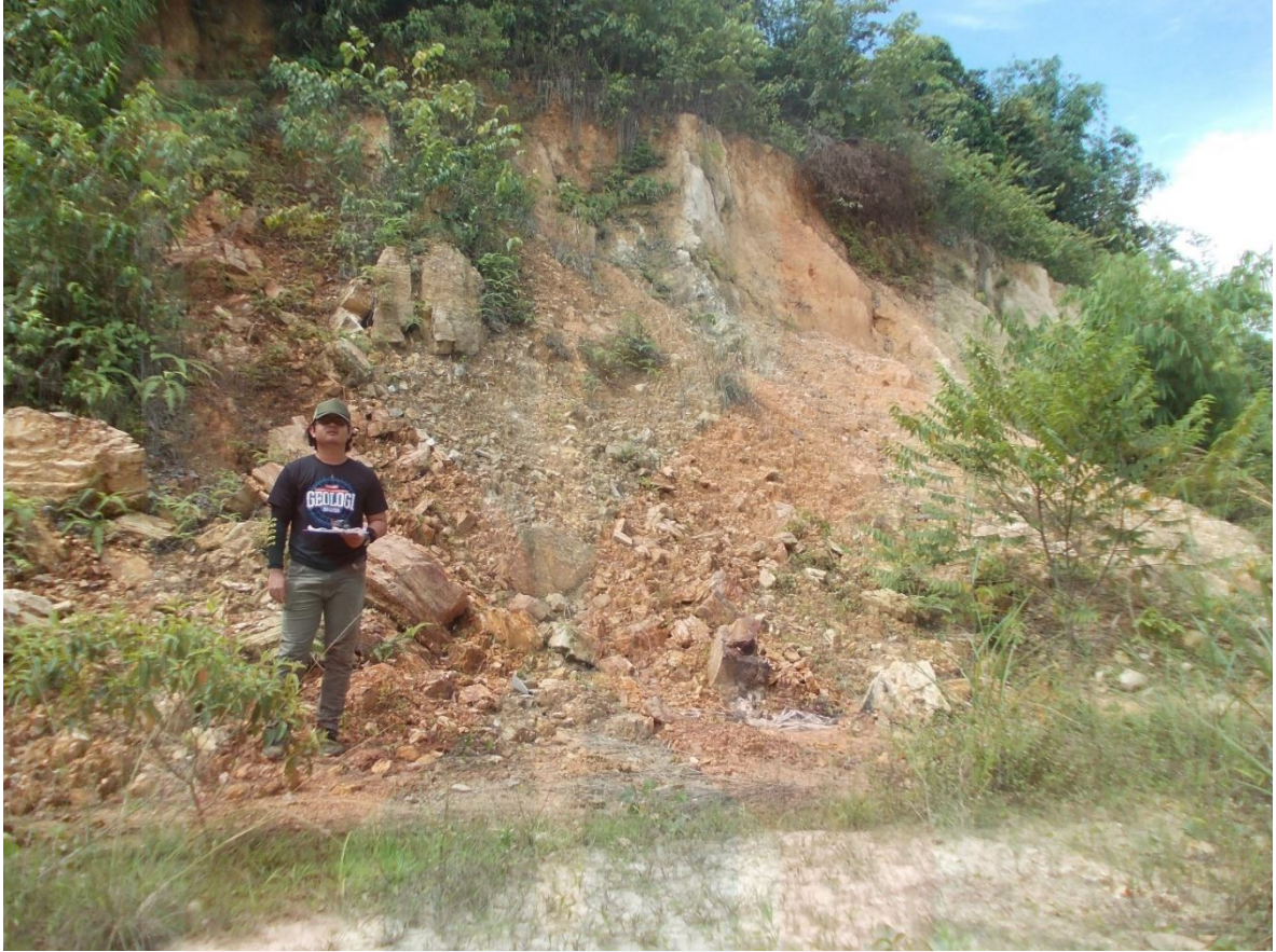
Figure 4.2: Mass Wasting (Landslide)
