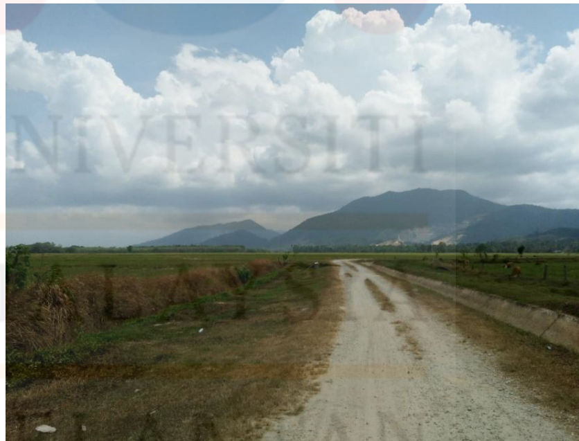
Figure 1.8: Unpaved road that connect the paved road with the plantation area
