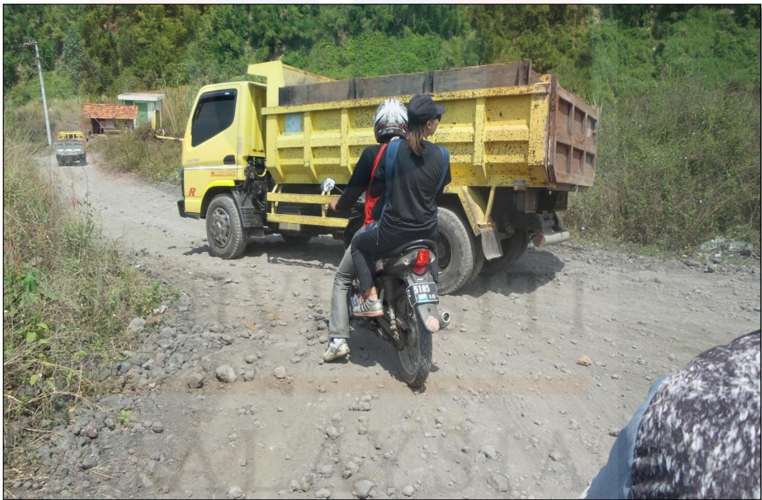
Figure 1.10 Road connection in Taragong area
