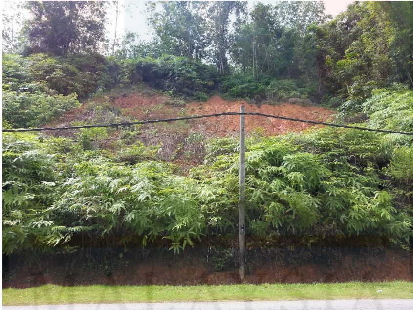
Photo E6: Slope failure 6
