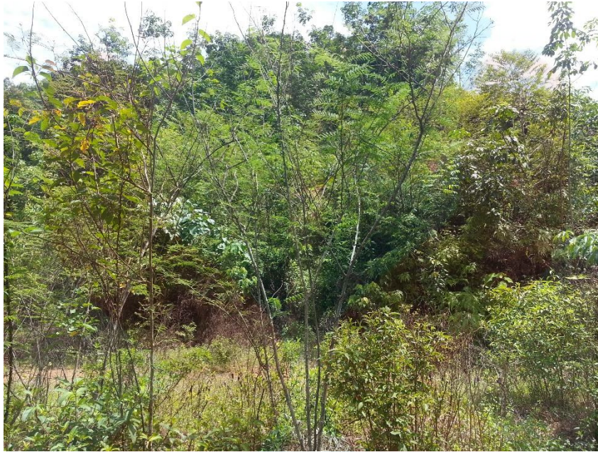
Photo E1: Slope failure 1 covered by vegetation (Coordinate: N 05° 24' 44.0", E 101° 55' 54.2")
