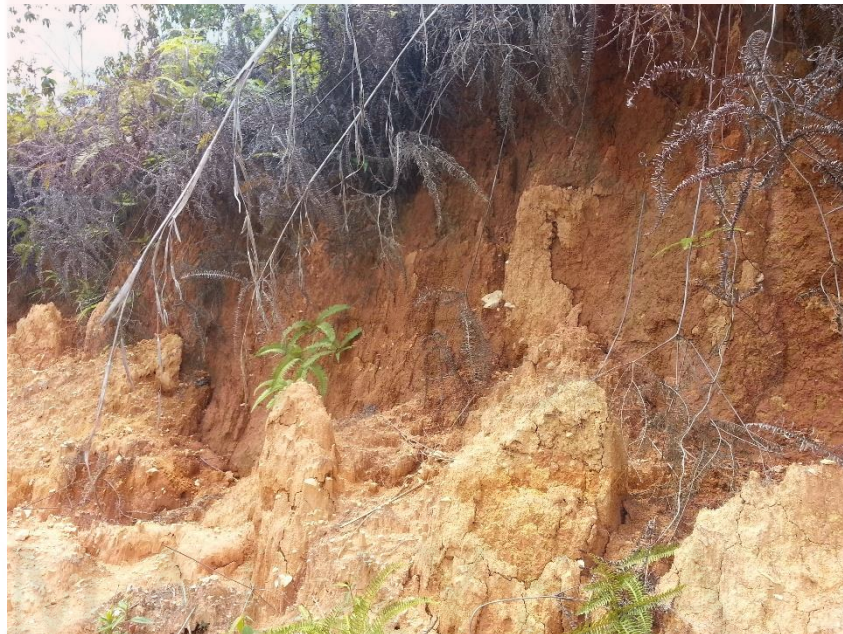
Figure 4.14: Gully erosion at 05°24'02.0", 101°56'47.0".
