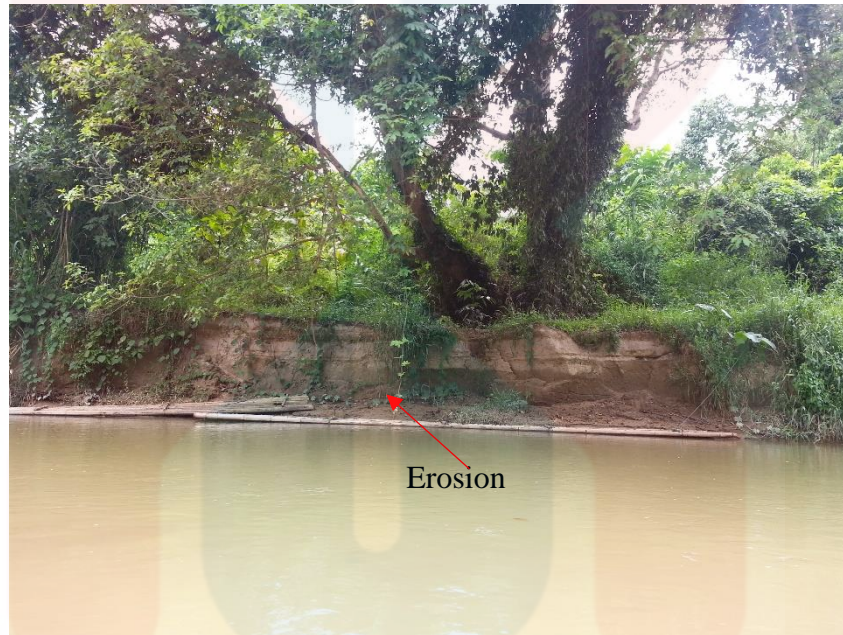
Figure 4.13: Erosion of river bank. (Coordinate: N 05° 25' 48.2", E 101° 56' 22.3")
