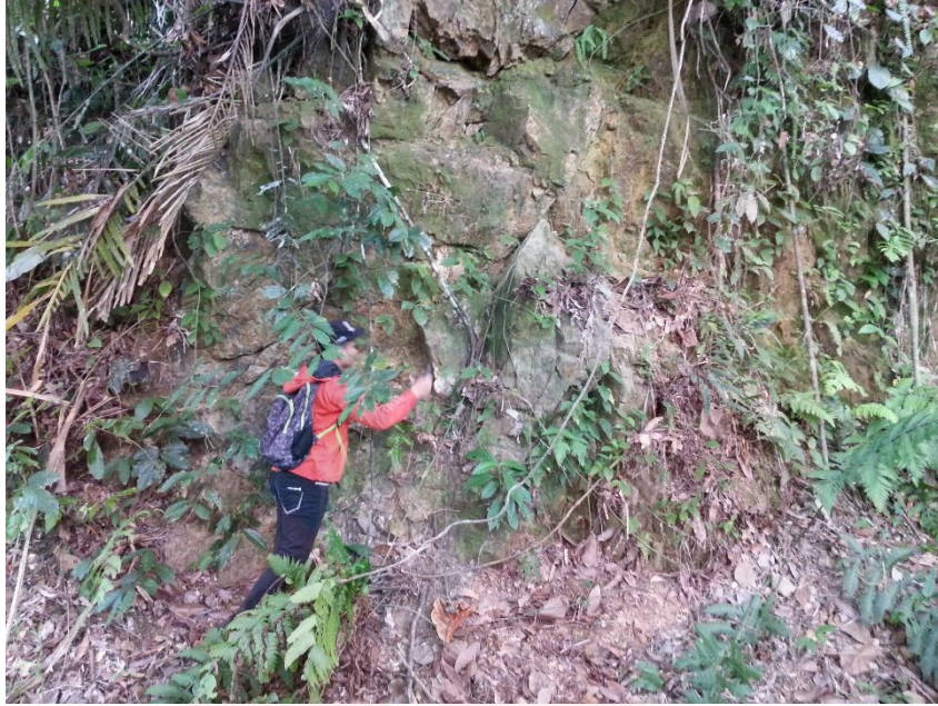
Figure 4.17: Root penetration by plants. (Coordinate: N 05° 25' 17.2", E 101° 54' 29.5")
