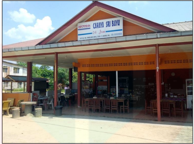
Figure 1.10: A 24-hours restaurant at Kampung Panglima Bayu
