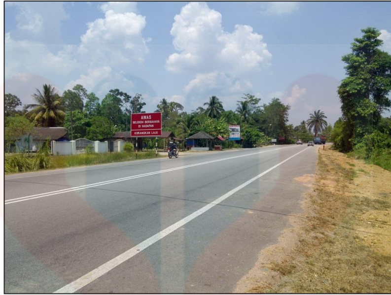
Figure 1.14: A part of the East-West Highway road
