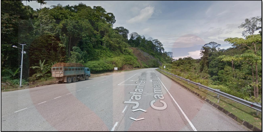
Figure 1.10 : The paved road in study area.
