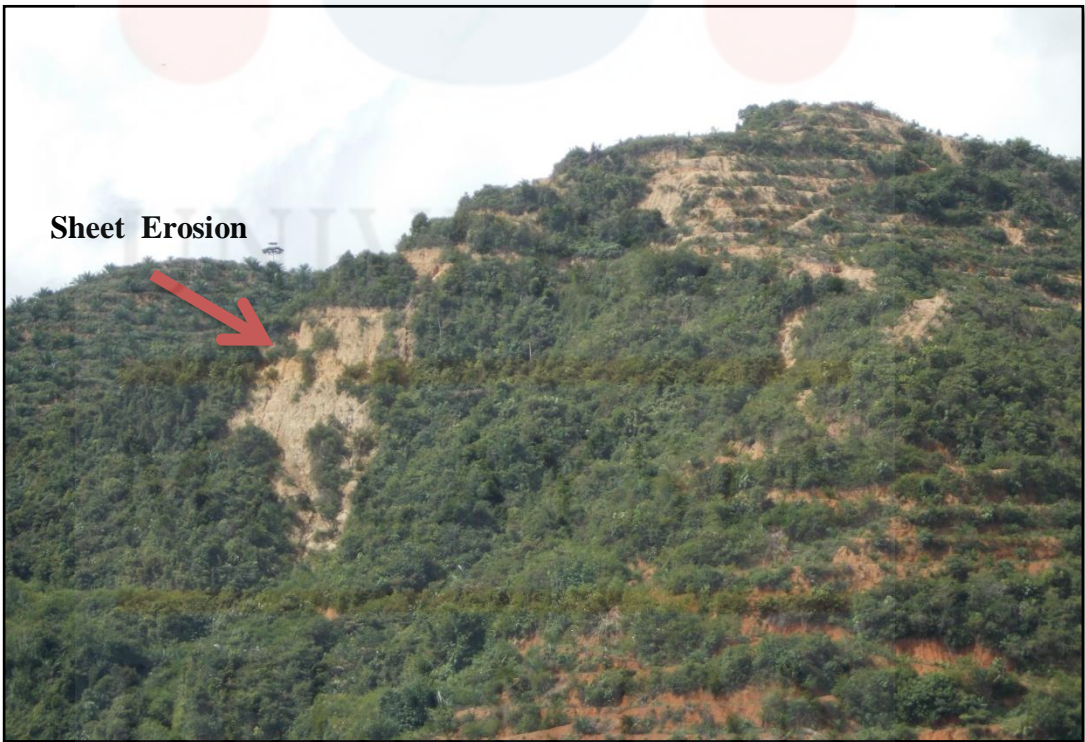
Figure 4.13 : Sheet erosion on hill in study area (red arrow)
