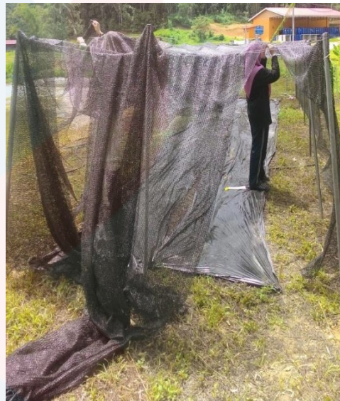
Figure A. 3: Shades area were constructed by paranet
