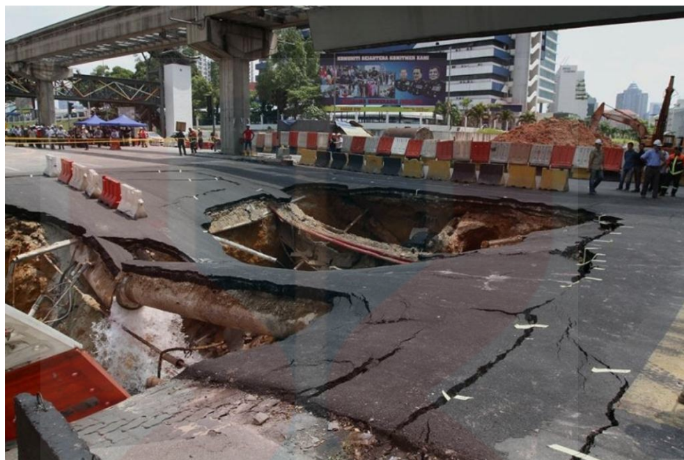
Figure 1.1 : A huge sinkhole caused by a burst water pipe is seen at Jalan Imbi in Kuala Lumpur, July 2, 2014. ( Source : The Malay Online )
