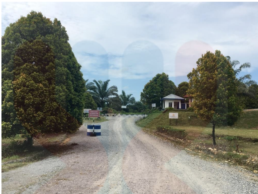
Figure 4.1: Road connection of Ladang Sungai Relai East
