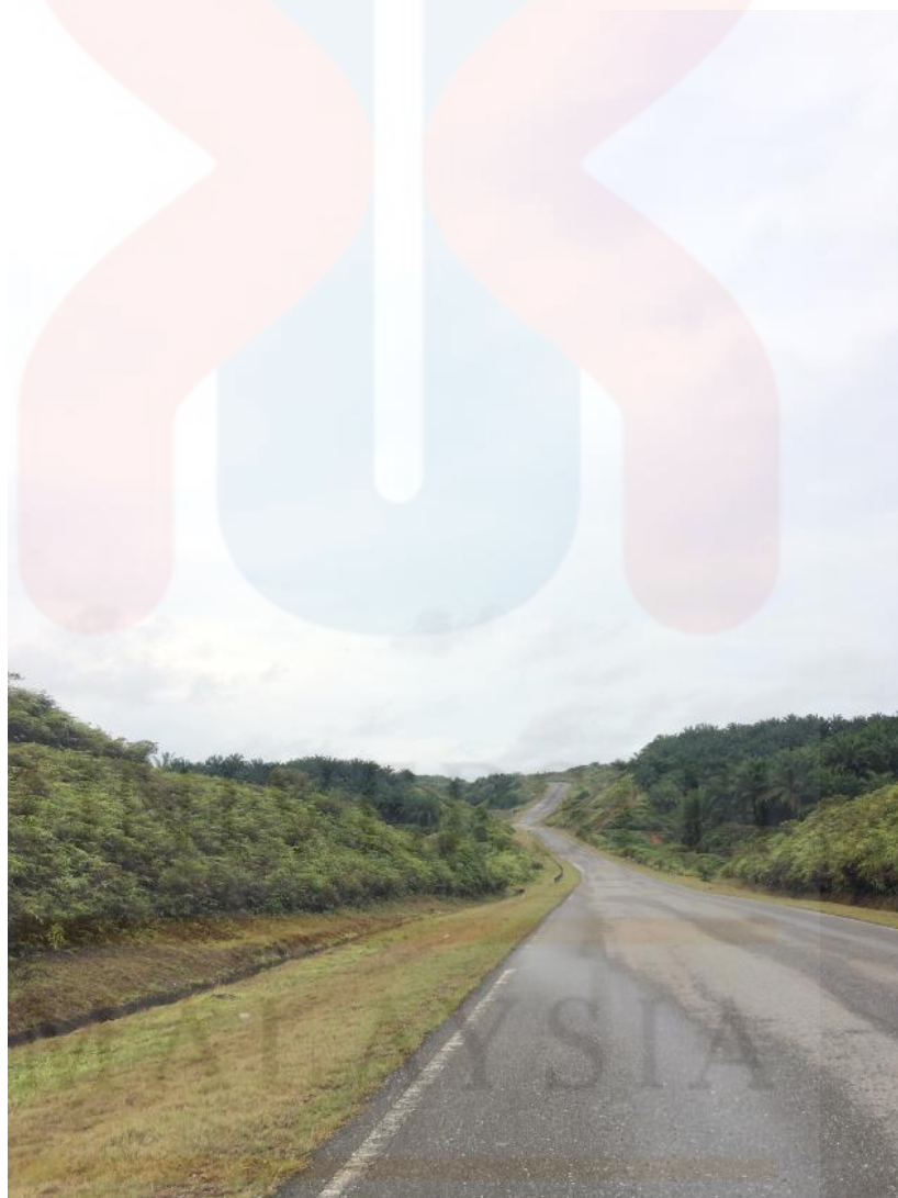
Figure 1.3: Main road connecting Kuala Berang (town) to Gua Musang (town).
