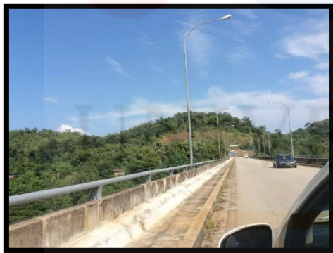
Figure 4.2: Dabong's bridge main road
