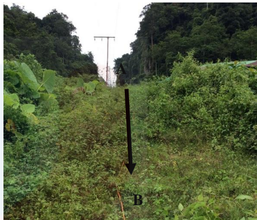
Figure 5.13: Line B in bushes area
