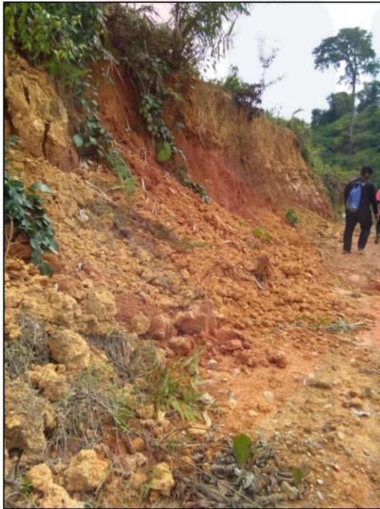
Figure 4.26: Slump type of mass wasting. Picture were taken with azimuth N 54 0 E at station 17.
