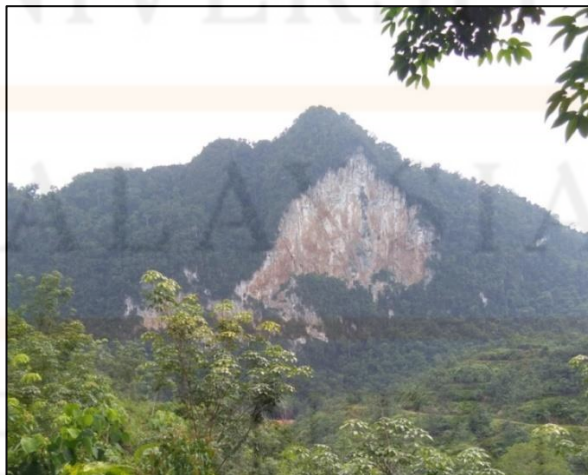
Figure 4.64: Scarp that has irregular shape on limestone wall.
