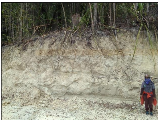
Figure 4.25: Biological weathering resulting of growth roots in crack of the rock. Picture was taken with azimuth S 26 0 W at station 2.
