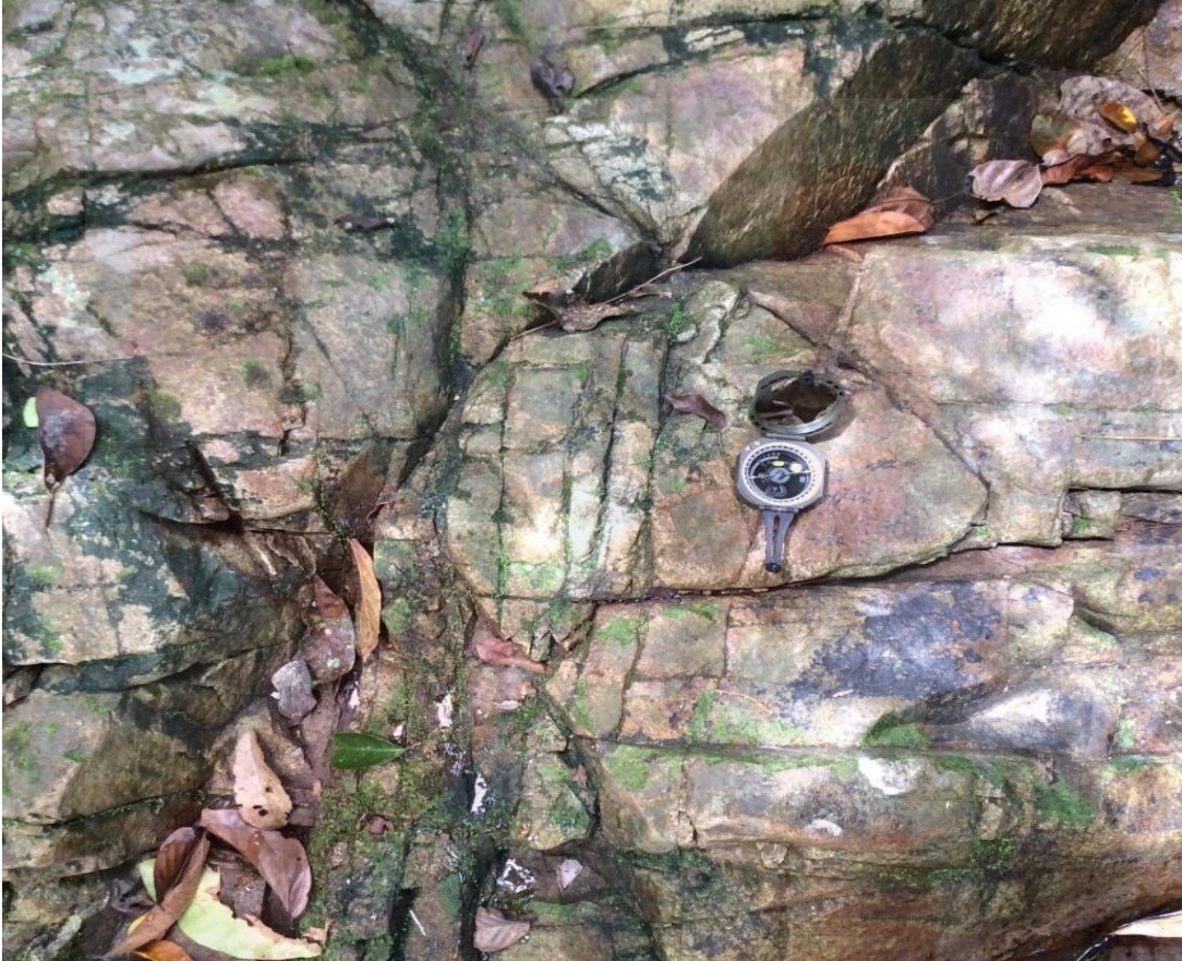
Figure 4.8: The joints at station 1
