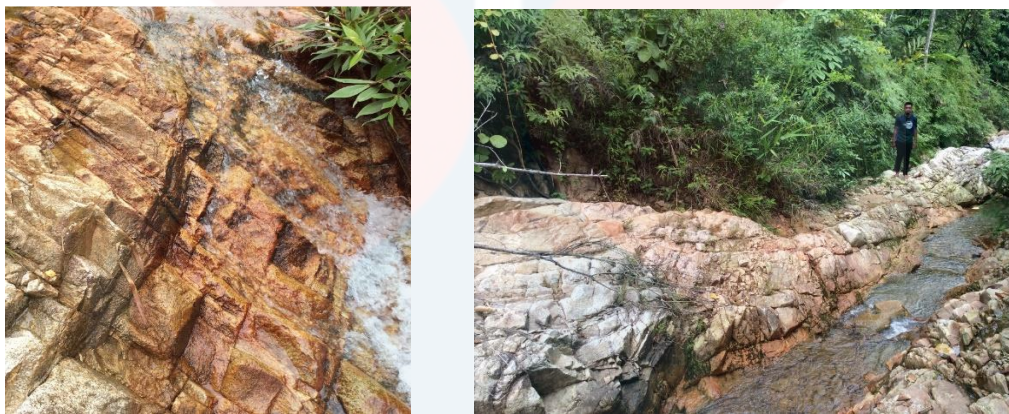
Figure 4.17 Great amount of shear joint
