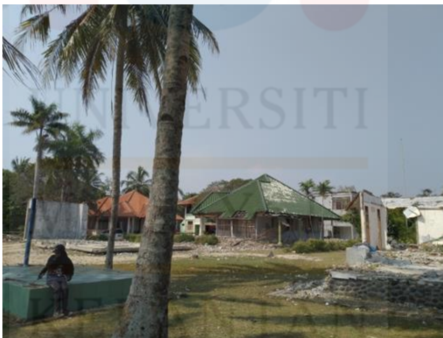
Figure 5.2: Villa that damaged due to the tsunami
