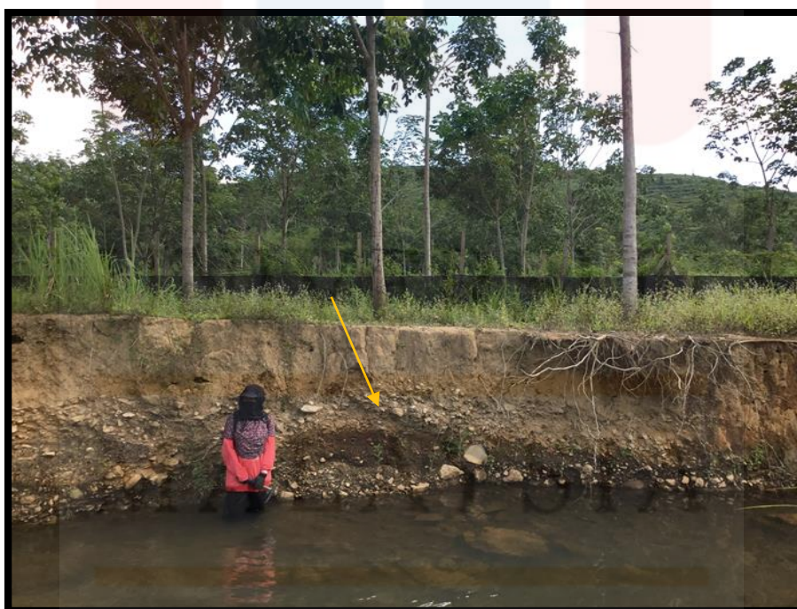
Figure 4.18 Showed the erosion of the river bank. (Coordinate: N 05° 43' 15.03", E 101°46' 2.22")
