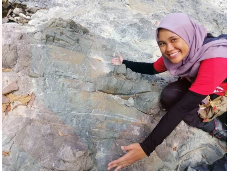
Figure 4.33: Sheeting joint found in Ngalang river at Nglanggeran formation.
