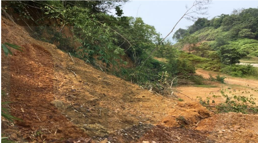
Figure 4.13: Minor landslide at N 05° 45' 15.3'', E 101° 44' 30.1''.
