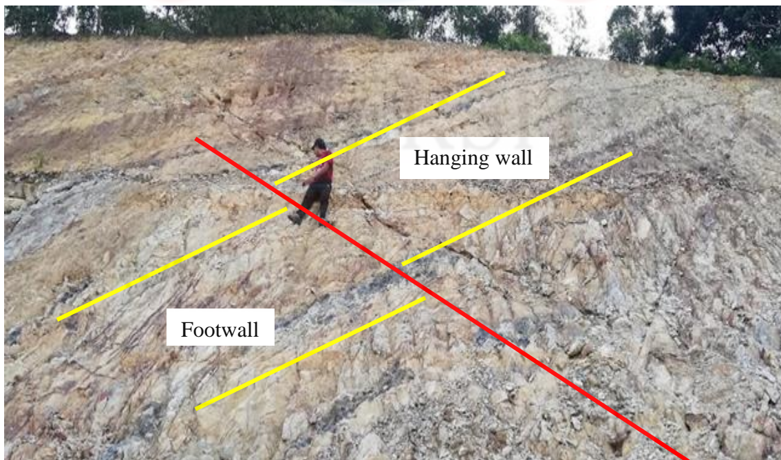
Figure 4.8.3: The Faulting (Reverse fault)
