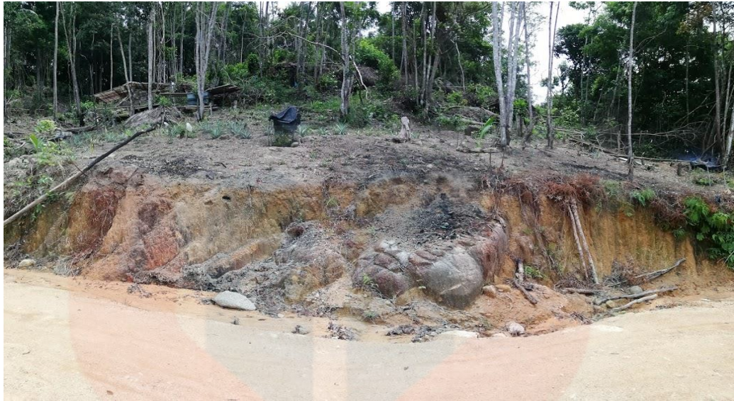
Figure 4.6.3: Slump type of mass wasting with coordinate of latitude 5.40511400 and longitude of 103.00763000
