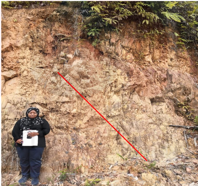
Figure A.2 : Minor fault
