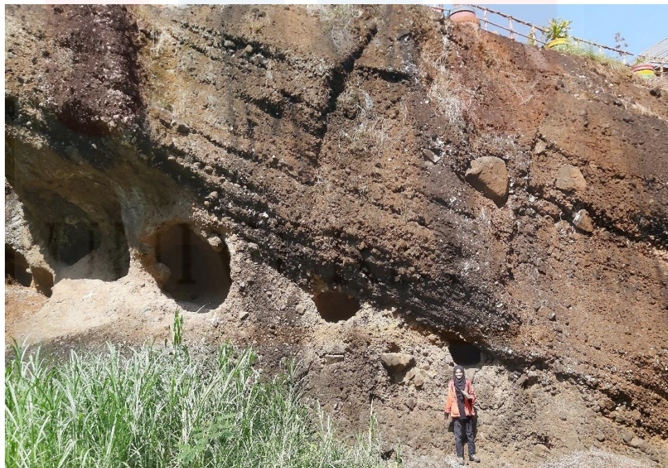
Figure 4.12: Example of Physical Weathering.
