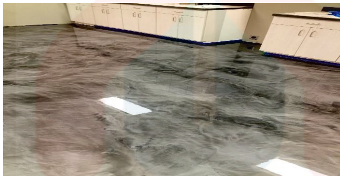
Rajah 1: EPOXY FLOOR COATING
