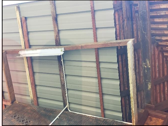
Rajah 5:2: Penambahan Metal Deck
