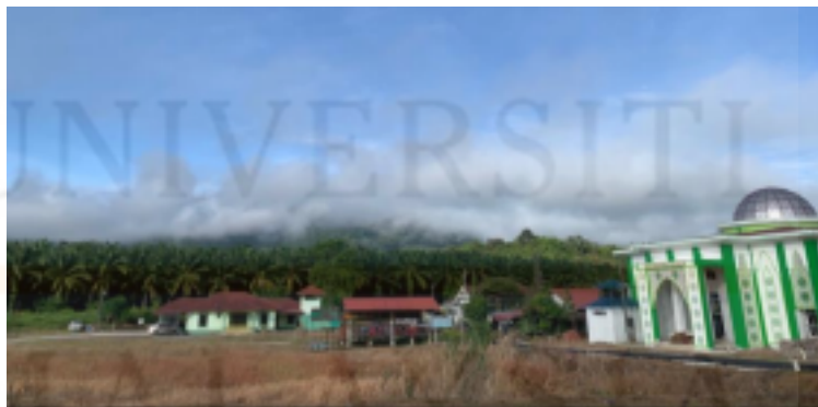
Figure 4.2 : Settlement at Kampung Kundur near to the main mosque of the village. (Coordinate: N 4° 52' 38.50", E 101° 56' 15.63")
