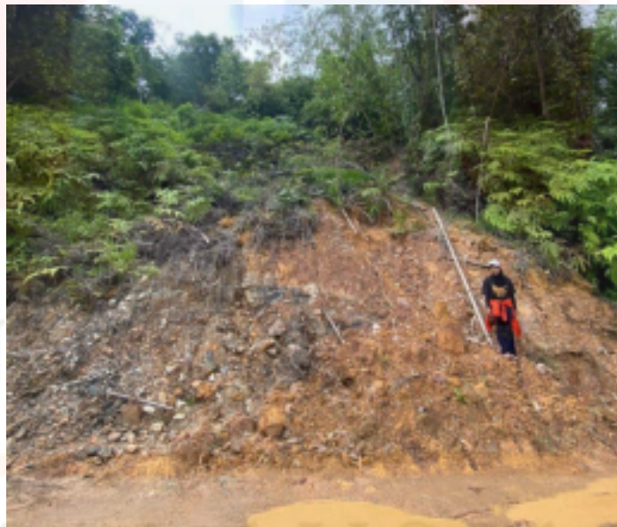
Figure 4.9 : Colluvium deposits at (a) roadside Jalan Dabong – Gua Musang; and (b) unpaved road near to Galas River.
