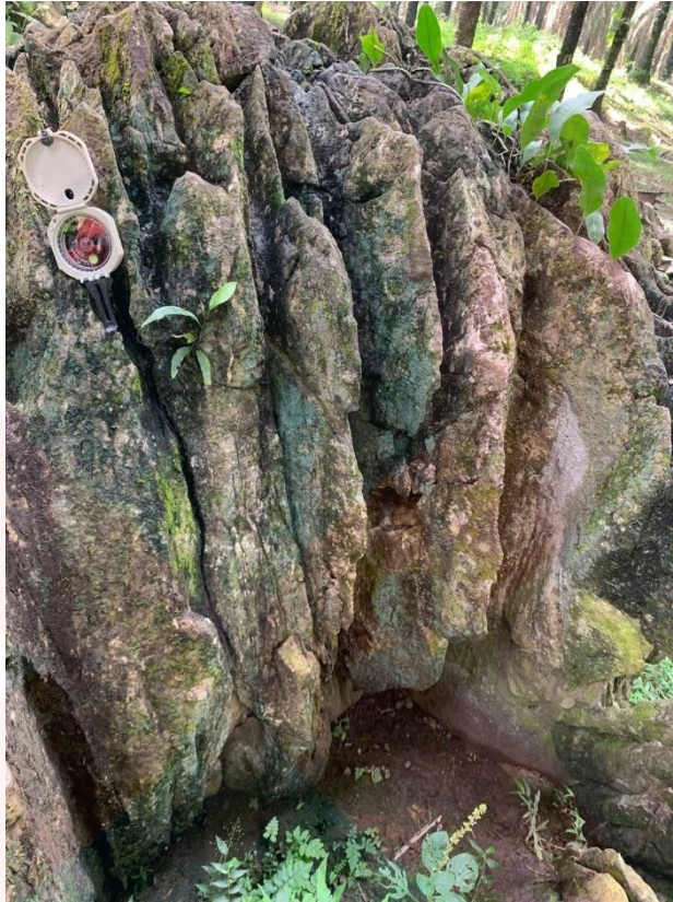
Figure 4.24: The picture of joint at station 13
