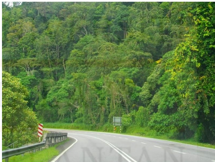
Figure 4.1 :The road connection of East-West Gerik Highway, Perak
