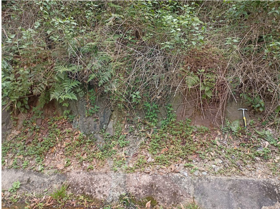
Figure 4.18: The outcrop that has joint discontinuities.
