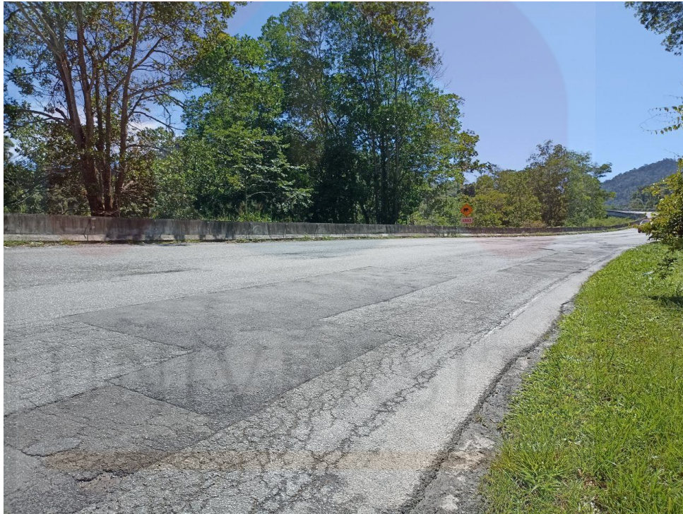
Figure 1.4: Road Connection between Gerik, Perak and Jeli, Kelantan.
