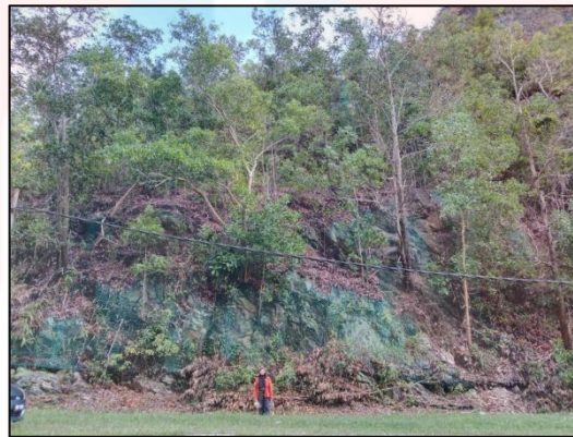
Figure 4.18 The condition of the first location.
