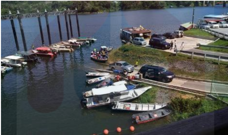
Figure 8 The situation at Banding public jetty.
