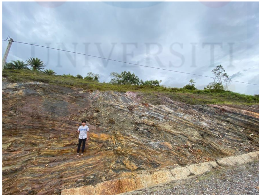
Figure 4.41 : Faulting that have in the study area .
