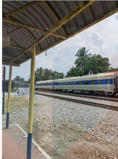
Figure 4.2: Railway track of Dabong
