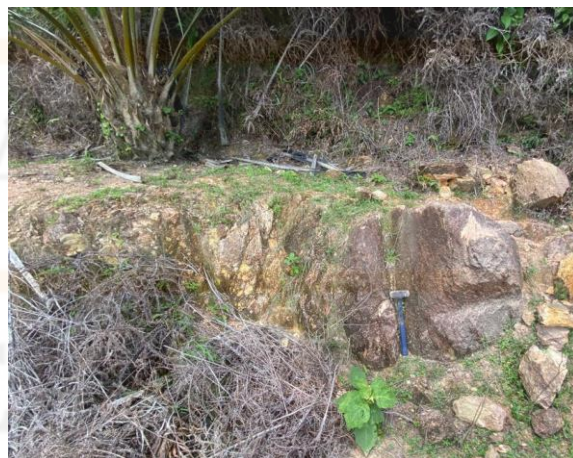
Figure 4.11: Biological weathering at study area.
