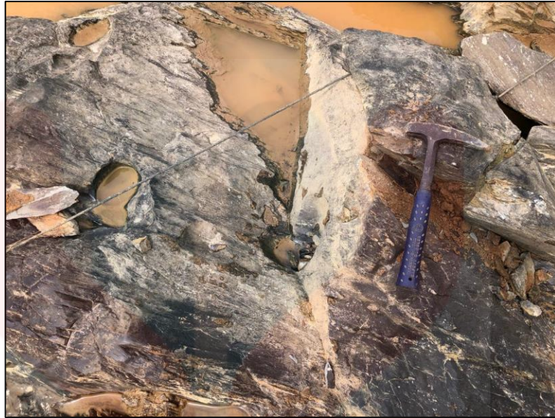
Figure 4.21: Joint structure on the slate rock.
