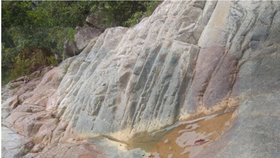
Figure 4. 19: Different shapes and orientations due to chemical weathering by rainwater and physical weathering by running water form a joint.
