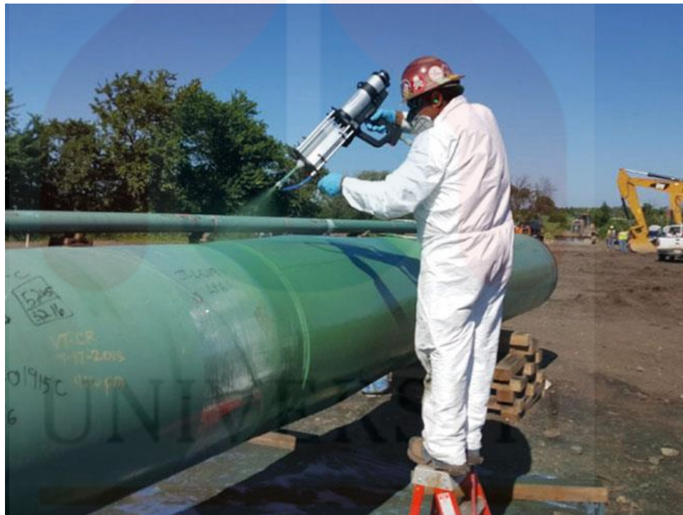
Figure 2.3: Epoxy coating application for welded steel
