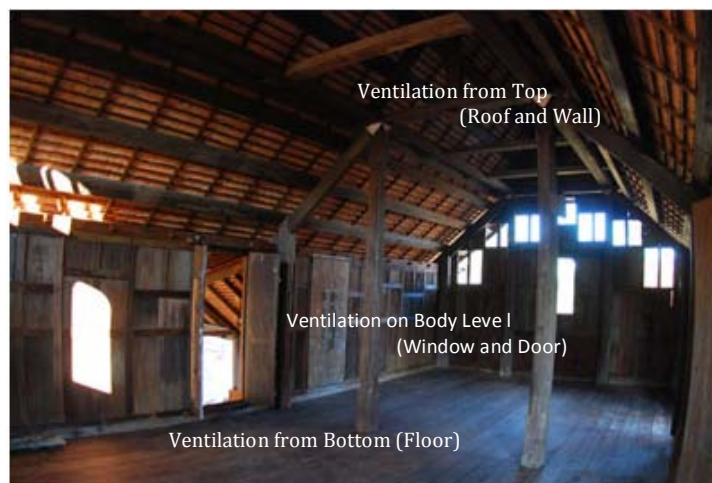
Figure 1.3: Concept of Ventilation for traditional Malay vernacular architecture.
