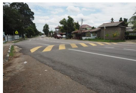
Figure 8 - Road Safety Measures or School Zone
