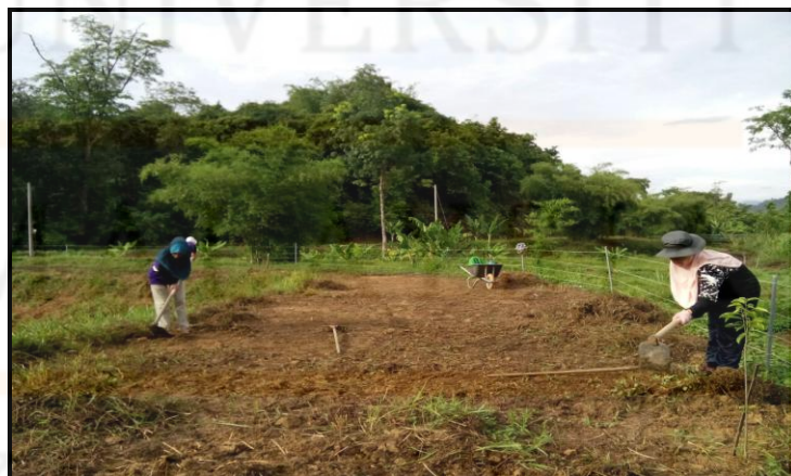
Figure 3.3 : Cleaning site process.
