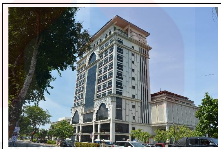
Figure 3.1: Image of Perdana Hotel.
