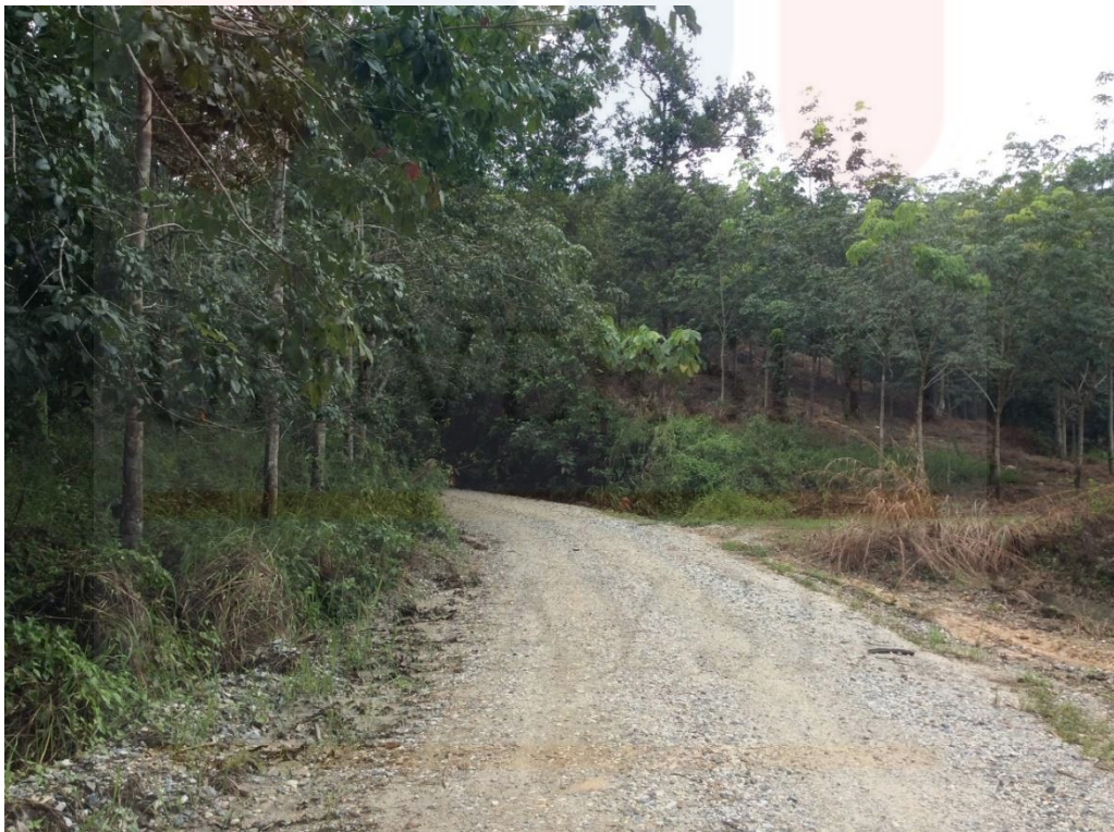
Figure 4.2: An unpaved road in the plantation area
