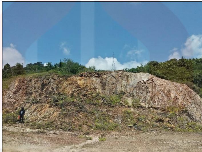
Figure 4.8: Example of outcrop that have physical weathering
