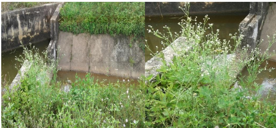
Figure 3.9 The place of sample collection at Kedah
