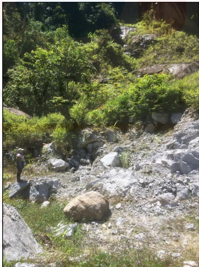
Figure 5.3. Slope failure in study area.
